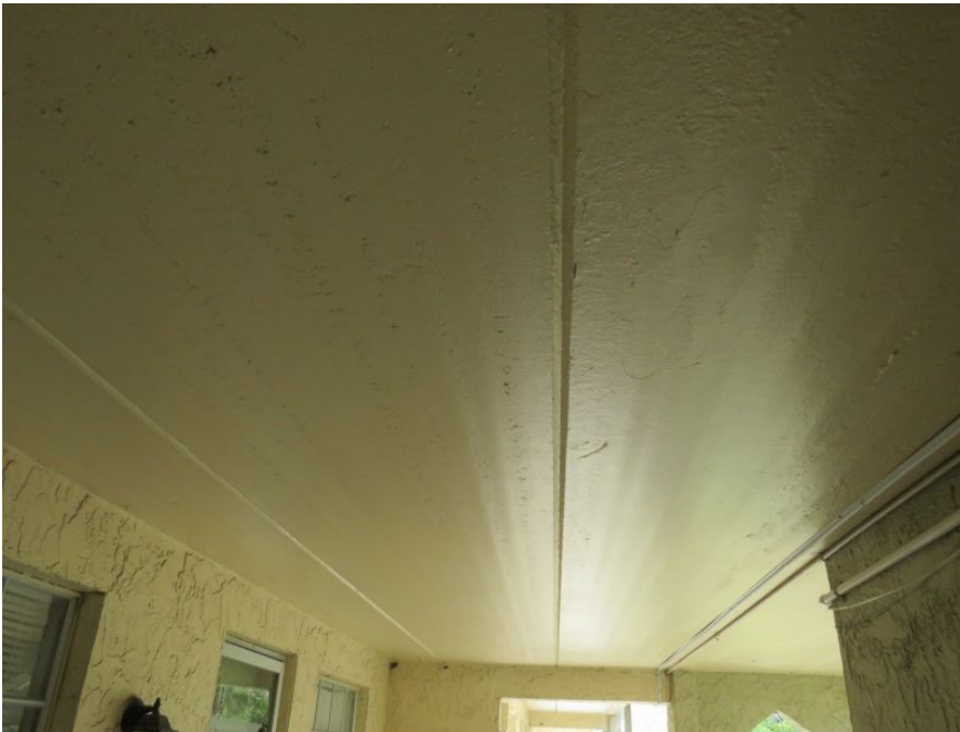
Reinforced Concrete Roof Deck
